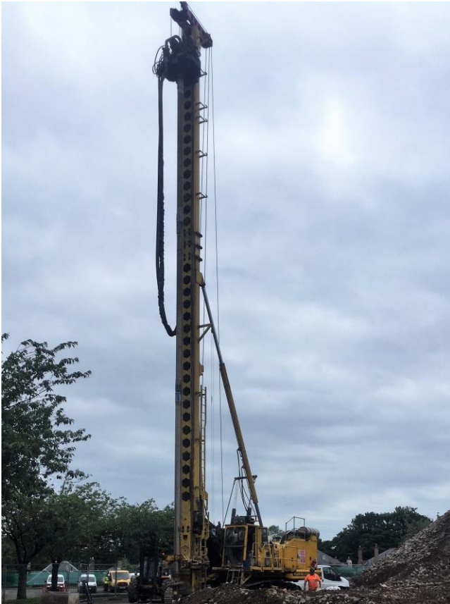
Picture 1: The Piling Rig arriving for the test piles
