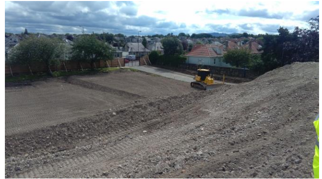
Picture 2: Ground works ahead of the piling mat
